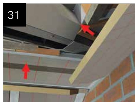
Fit 25mm insulation.
