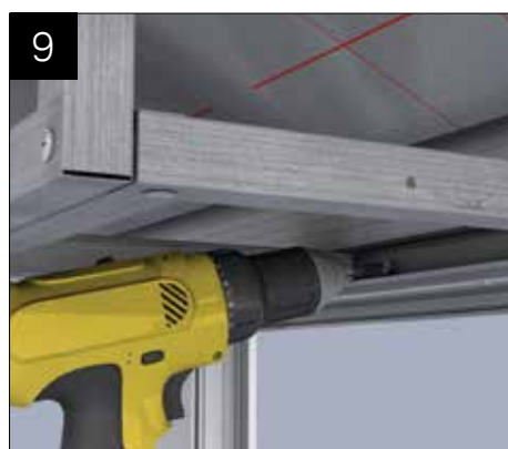
CHA008 4.8 x 32 Self Drill Philips Pan Head
