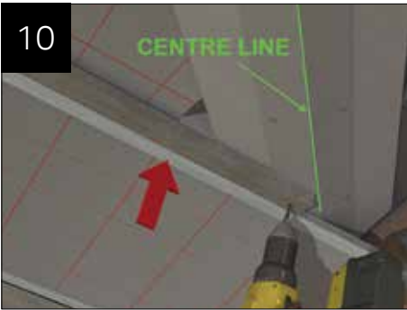
Fit the ridge battens, as described on page 39. NOTE: On the valley side, the batten should terminate on the valley Plate centreline as shown.
